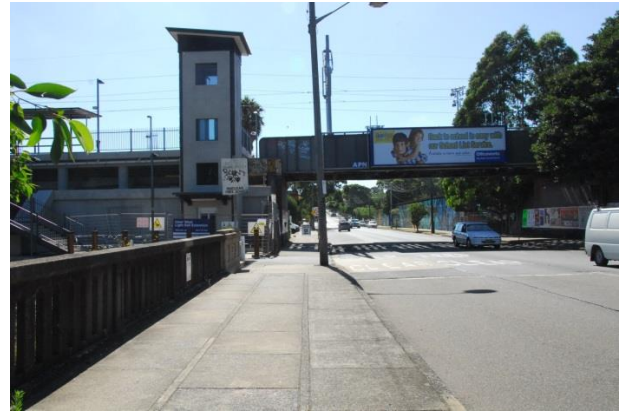
Figure 11: Marion Street – view east to railway overpass/bridge and light rail stop
